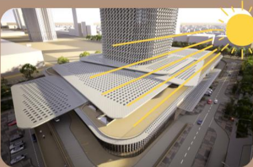
SKYLIGHTS COVERED WITH PERFORATED ROOF
