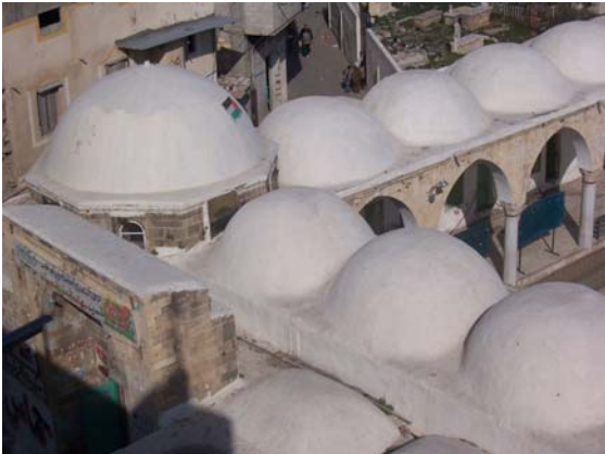
Fig. 4. The Semi-spherical roof domes of Al-Said Hashim Mosque.
