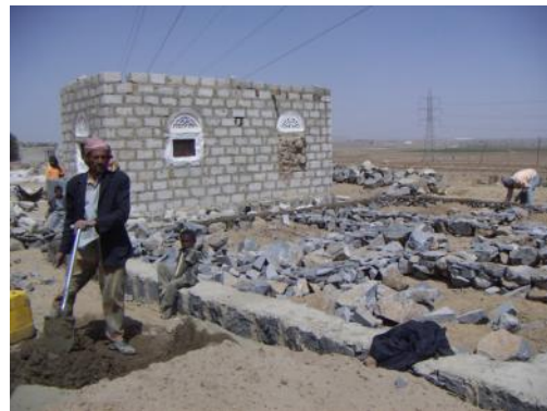
Fig. 10. The construction of a '1,000,000 YR house' in Dhamar with the help of an informal contractor. Unfortunately, the house is built along the city fringe on an unplanned (cheap) plot of land that is very close to a power line.
