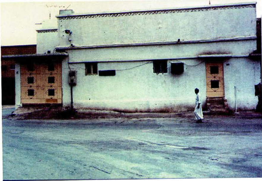
Fig. 7. A photograph of one of the transitional houses shows the character of transitional architecture of where cement blocks and plaster are the main building materials replacing adobe.
