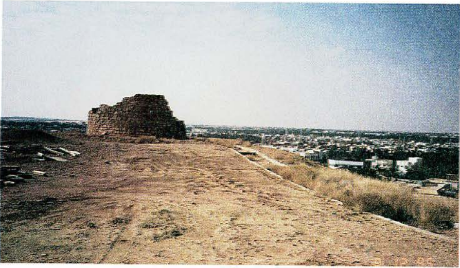
Fig. 7. Al-Sungar is a Turkish name for warning and defense tower. c Onaizah town had two sungars which were built of stone and constructed on eastern borders of the town. One sungar was demolished but redesigned with the whole cultural center of Saleh Bin Saleh while the ruins of the other one remained waiting for remodeling.
