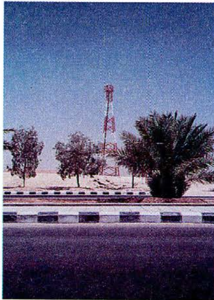
Fig. 18. Telecommunication towers replaced functionally the warning and defense towers but the technology influenced their form and height.
