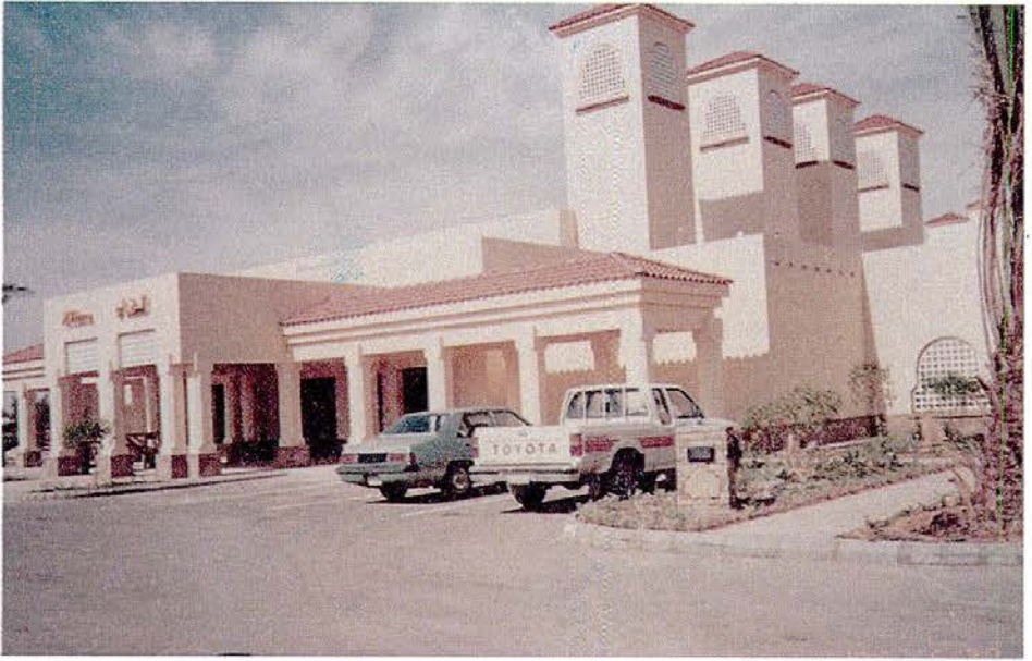
Fig. 23: The wind tower is associated regionally with the Arabian Gulf region. The building of the Gulf consolidated countries in Riyadh took the tower as an icon for the building.
