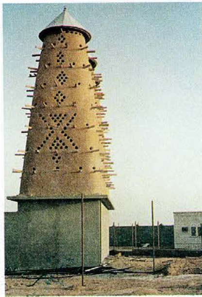
Fig. 19. The domestication of pigeon and doves necessitated the building of towers which serves as a good ventilated and secured space for pigeons.
