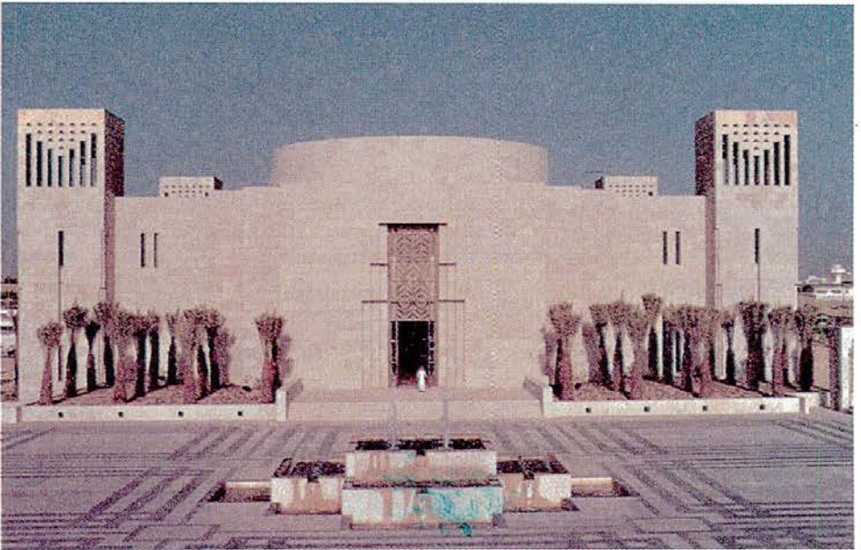
Fig. 24: The photograph shows four Malqafs (cooling towers) recently built in Al-Nozl (Hotel) in Skaka town in Al-Jouf region north of Saudi Arabia to ventilate closed onopen spaces.
