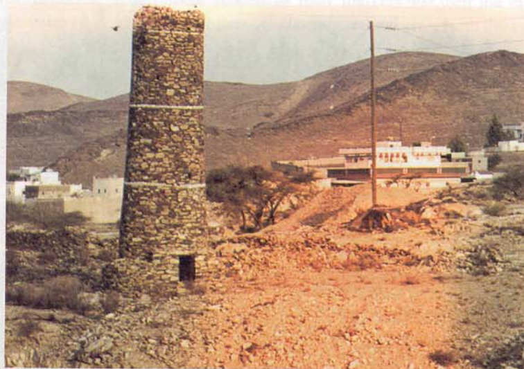
Fig. 10. Al-Qasabah is the synonym given to the “warning and defense tower” in the southern parts of the highlands of Saudi Arabia.
