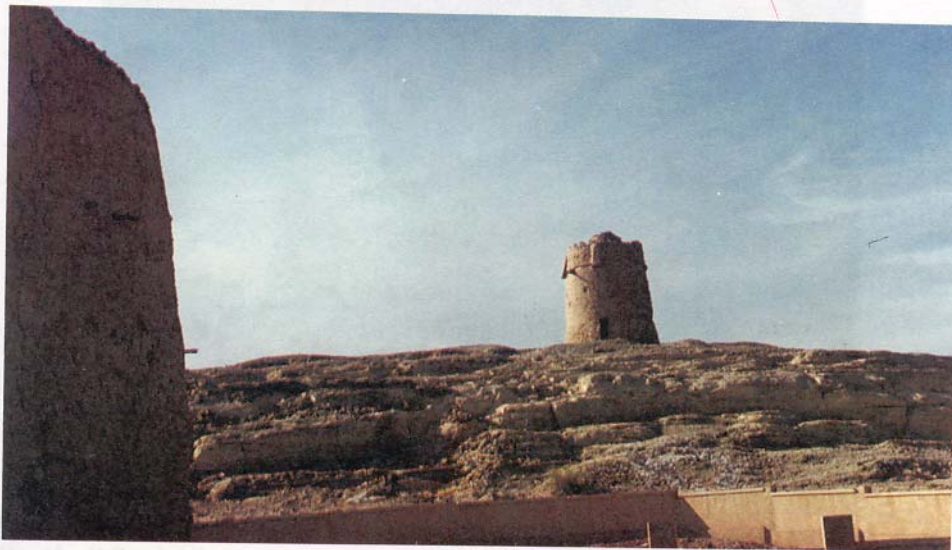
Fig. 7. Al-Burj is the synonym given to the "warning and defense tower" in the central parts of Saudi Arabia.
