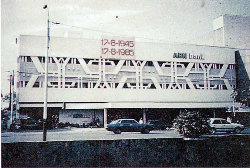
Fig. 12. An example of a wall design utilizing contrast between plain and textured walls.
