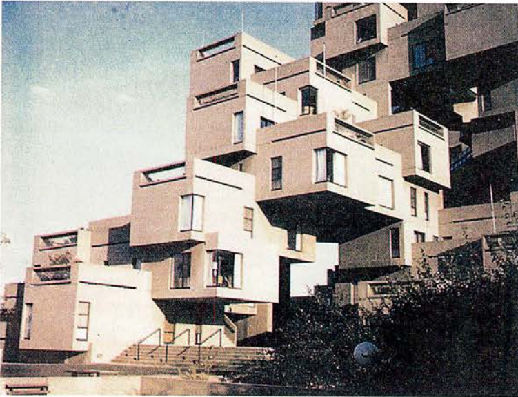
Fig. 14. Housing in Expo 67 designed by Mose Safadie, an example of interlocked multiple rectilinear form [23, p. 387].
