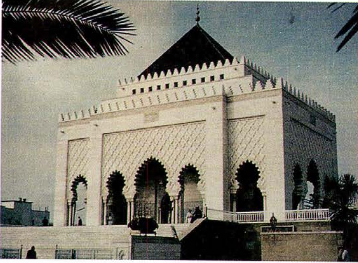
Fig. 6. The Mausoleum of King Hassan II in Rabat, Morocco, an example of recessed walls.
