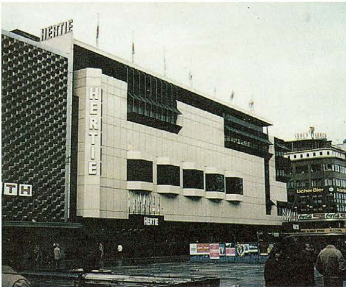
Fig. 11. A commercial building in Frankfurt, Germany. This is an example of a relief wall, where flat areas are contrasted with projections or cavities.
