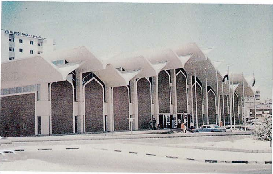
Fig. 5. An example of roof dominated building, full enclosure: Sharja (UAE) Post Office building.
