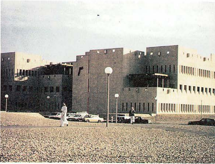
Fig. 13. Typical King Saud University buildings, an example of multiple rectilinear form.
