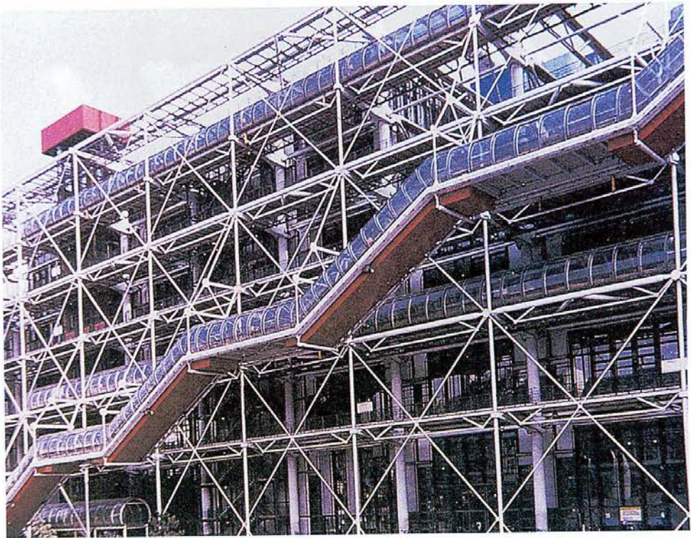
Fig. 8. The Pompidou Center in Paris by Richard Rogers and Renzo Piano, a wall dominated by non-enclosing elements (mechanical and structural) [16, p. 375].
