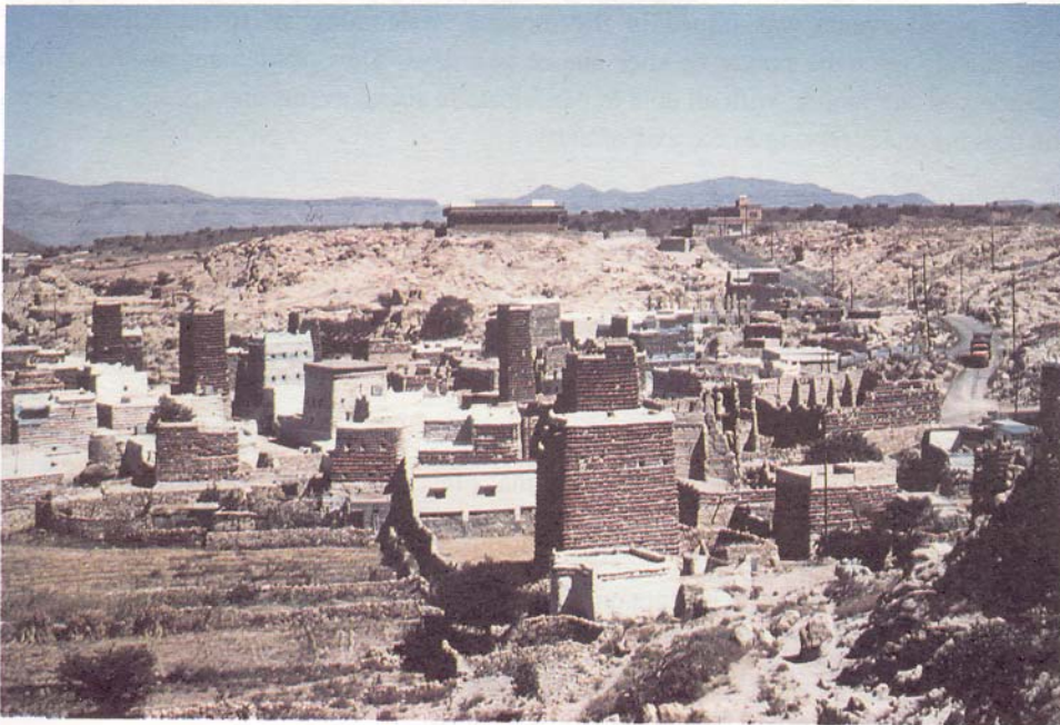
Fig. 4. The southwestern mosque, the second mosque built on the periphery of Al-Alkhalaf, is distinguished from a distance by its form, color and height.
