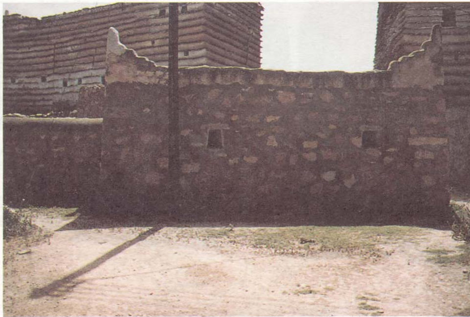
Fig. 8. Exterior of Al-Masjid Al-Jamic showing the openings on the eastern facade and the architectural characteristics of the mosque.
