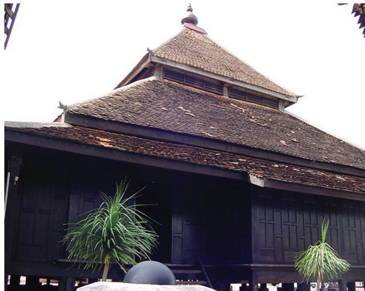
Figure 2: KLOM with its triple roof form.
