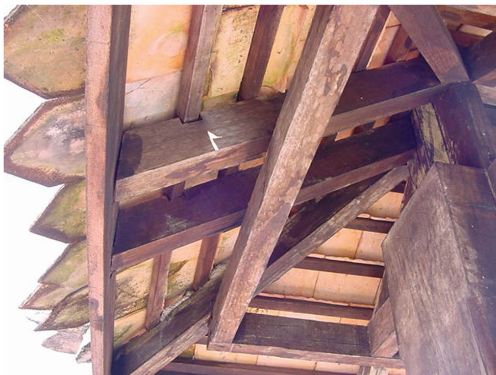
Figure 3: A roof covered with Senggora roof tiles.
