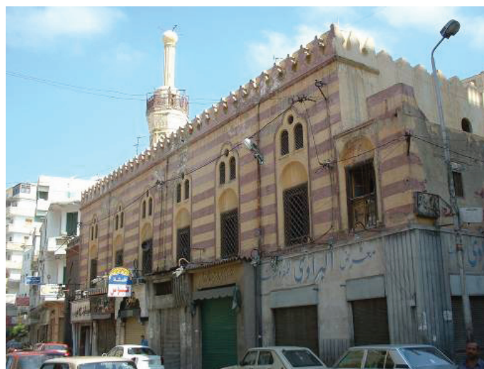
Figure 13: Terbana Mosque. The ground floor is used as shops while the praying area is raised to the upper floor
