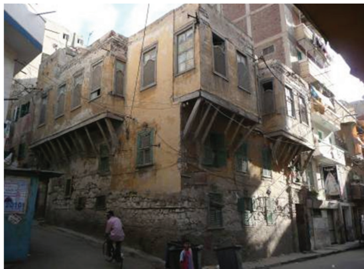
Figure 5: Typical house of the Ottoman Town. The second floor overhangs to the street, supported by diagonal wooden bracings. Openings are screened to control light and provide privacy
