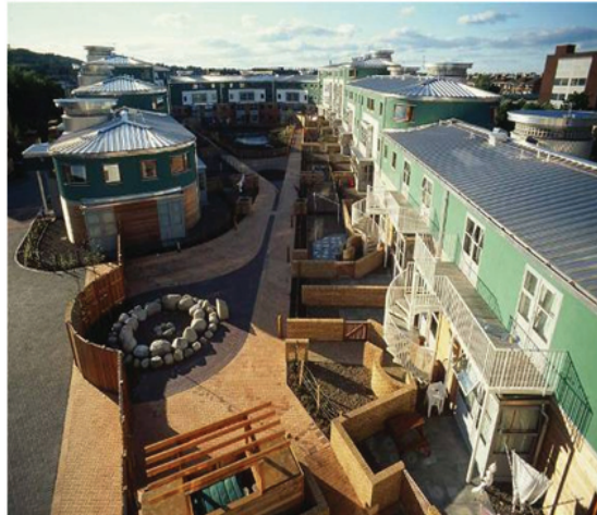
Fig.11: Terraced Gardens which Surrounded by Natural Landscape and the Inner Pedestrian Walkway [18].
