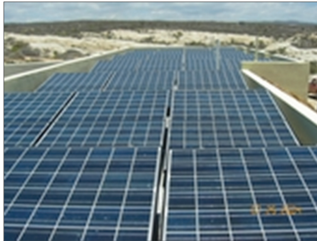
Figure 4: Solar Panels as an Addition to Existing Building.
