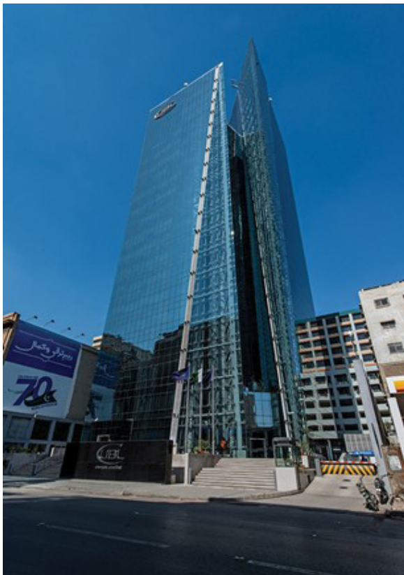
Figure (9). The 23 stories UBL tower completed in 2016 in Karachi
