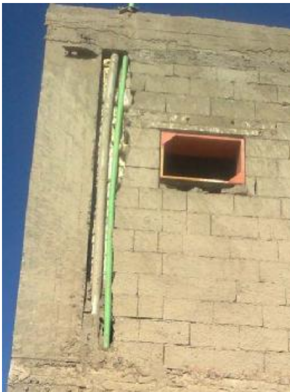
Figure 2. Two services (Sewage and water pipes) introduced at end of the beam and column's interior face breaking the wall's bond with the column.
