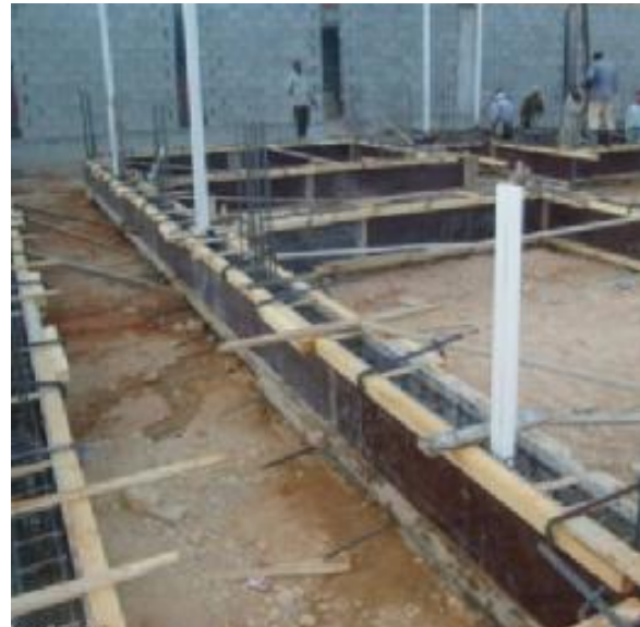
Figure 3. Introduction of pipes at several points across the depth of ground beams.
