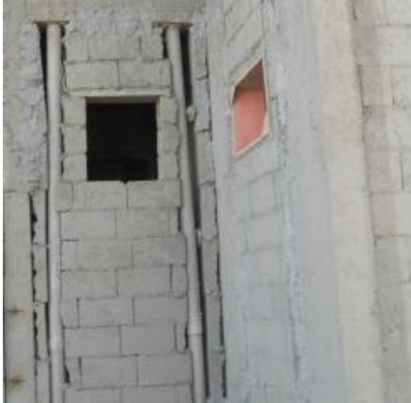
Figure 1. Sanitary pipes passing across the depth of the beam and across the wall's height
