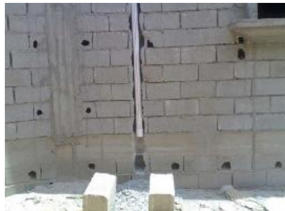
Figure 4. Beams showing the exposure of the reinforcement due to introduction of pipes across the depth of the beam.
