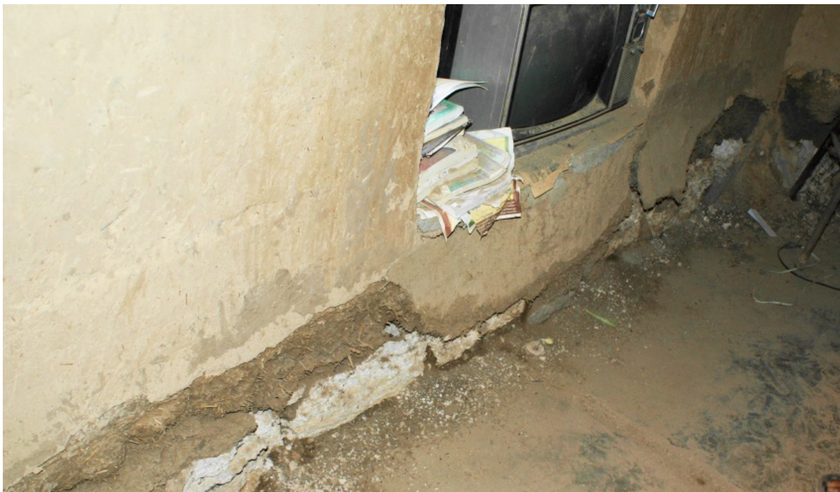
Figure 2. The walls inside one of the earthen houses in New Gournia have deteriorated dramatically due to the infiltration of the rising dampness and rising ground water level and the lack of adequate damp insulation, as shown in this photograph. Inadequate restoration work carried out to these walls have even worsened their condition (the author).
