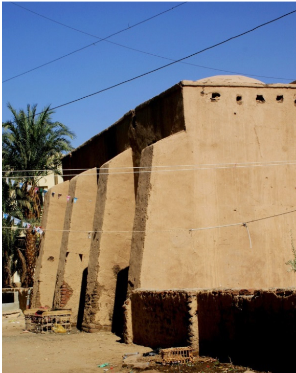
Figure 13. The four buttresses that have been added to one of the side walls of the theatre during the conservation works carried out by Hassan Fathy (the author; Moustaaader, 1985).
